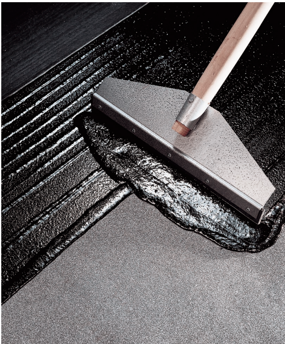
Applying DERBIBOND S with a toothed roofer's squeegee.
